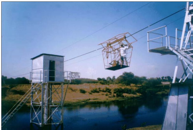
Figure 6.30: Cableway with manned trolley
